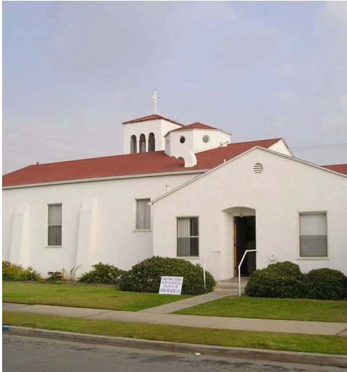
All was ready at the corner of Carson & Gardenia.
